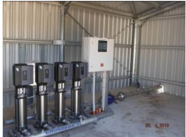
Photo 22 – LG Bore Transfer Pump Station
