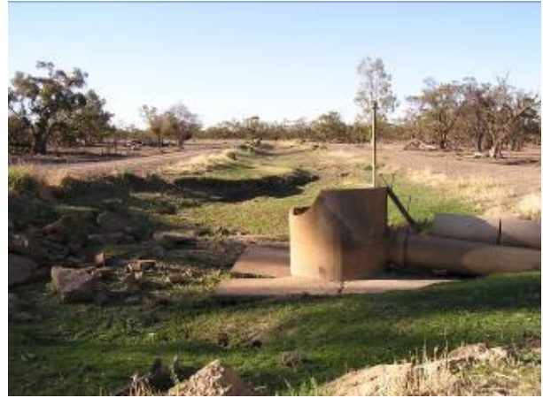
Photo 26 – NWA Channel Stilling Basin
