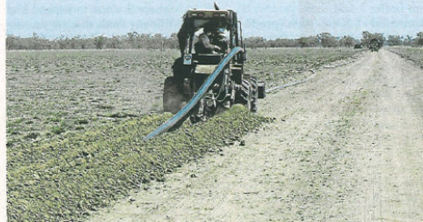
Aquawest crews from Dubbo have been busy working on a pipeline to supply landholders with Barwon River water. Work at the southern end of the pipeline has involved digging trenches to carry 125 millimetre pipe.
