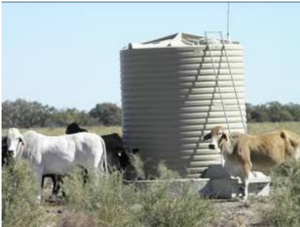
Photo 17 – Cup & Saucer Tank on BCA project
