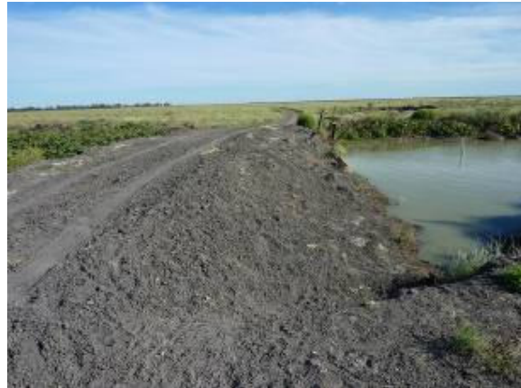
Photo 6 – Narran Channel Block Dam to Stop Breach
