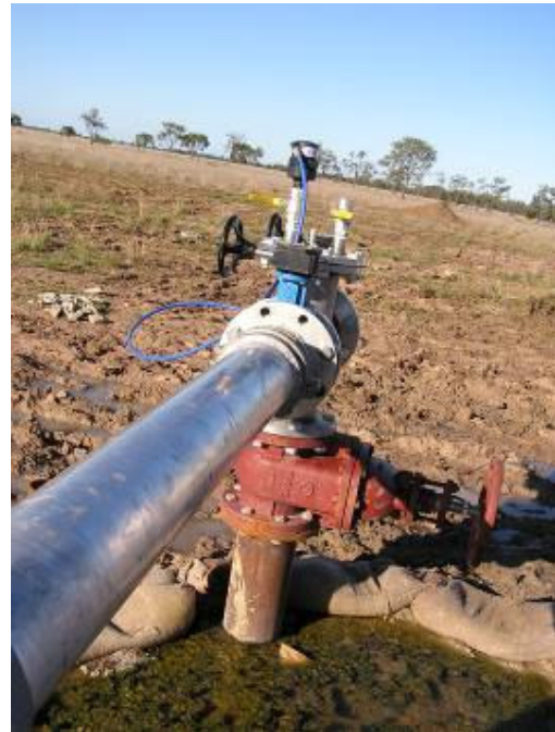
Photo 8 – GAB Bore GW 273148 sunk to 206m
