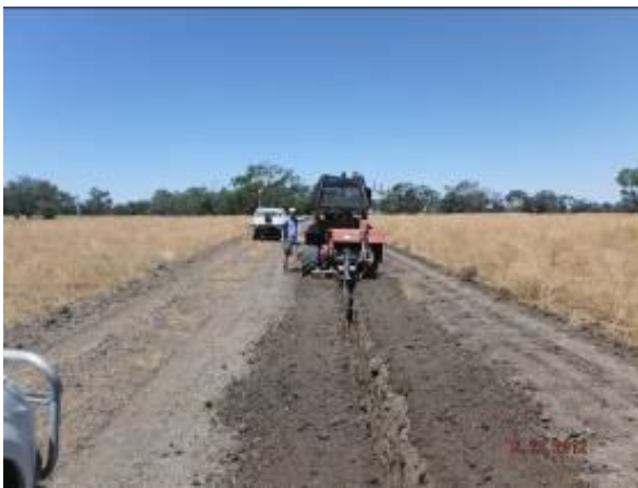
Photo 23 – Pipe Trenching on LG project
