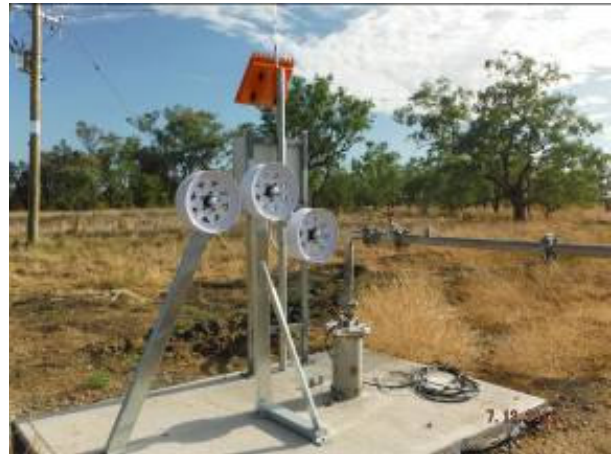
Photo 20 – Bore Headworks on LG Project
