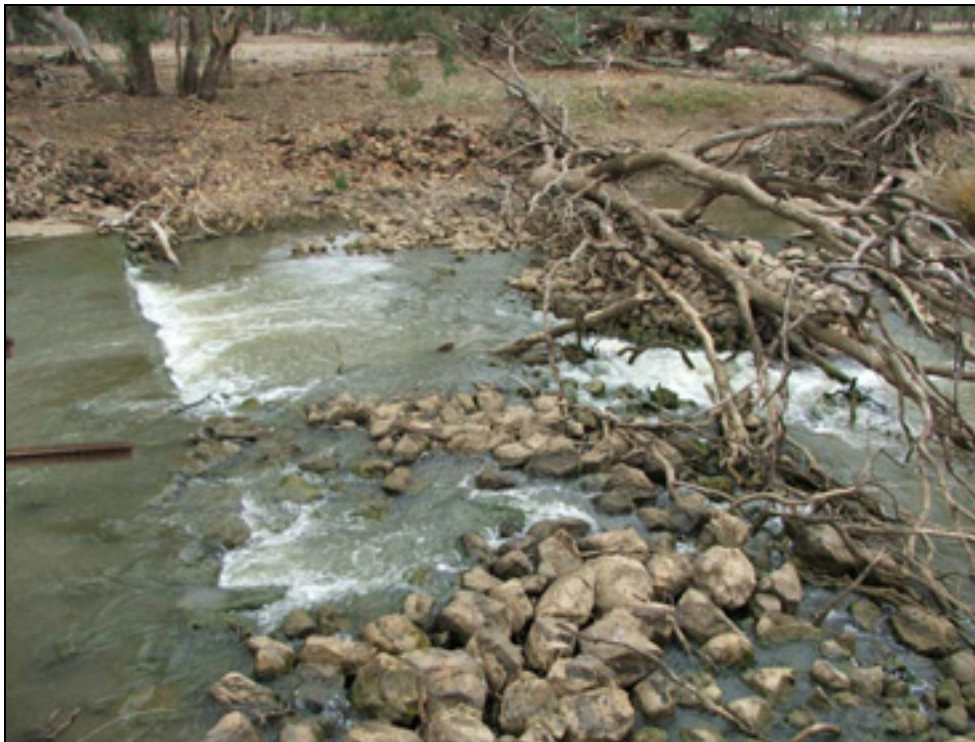
Figure 2. Kennedy's Weir, rock spillway, Goobang Creek (28.04.2005, 95ML/day).
