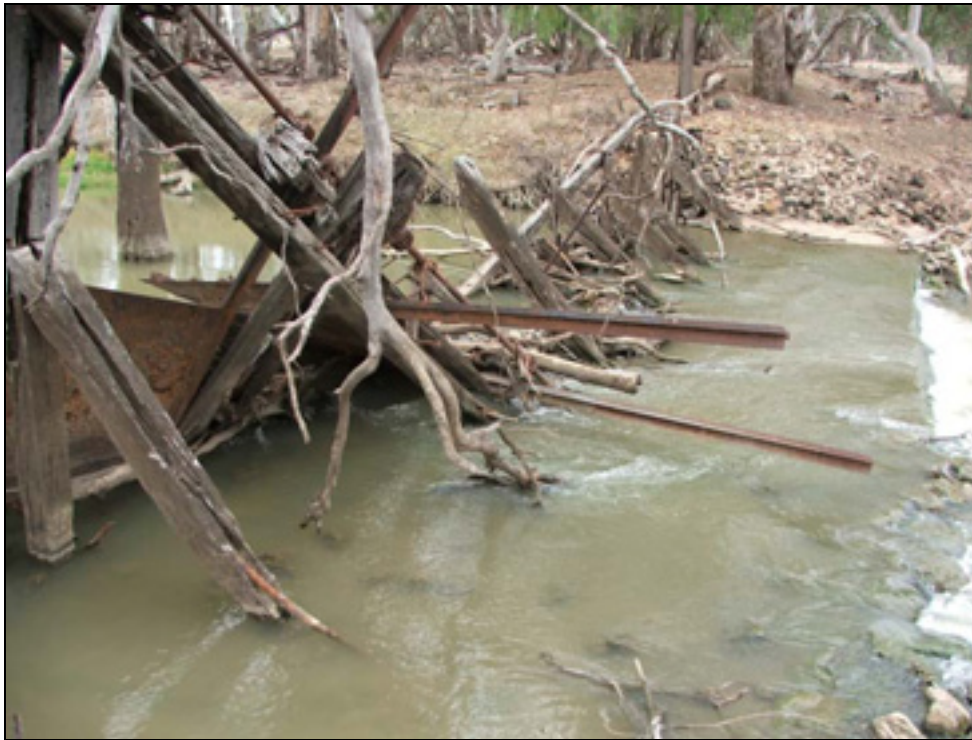
Figure 1. Kennedy's Weir defunct regulating structure, Goobang Creek (28.04.2005, 95ML/day).
